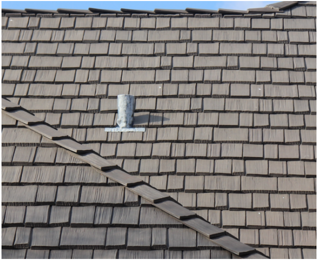
Example #5: Synthetic Cedar Roof
