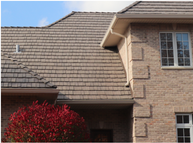
Example #5: Synthetic Cedar Roof
